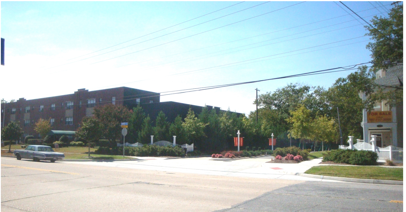
“BEFORE” : RIVERSIDE TERRACE
